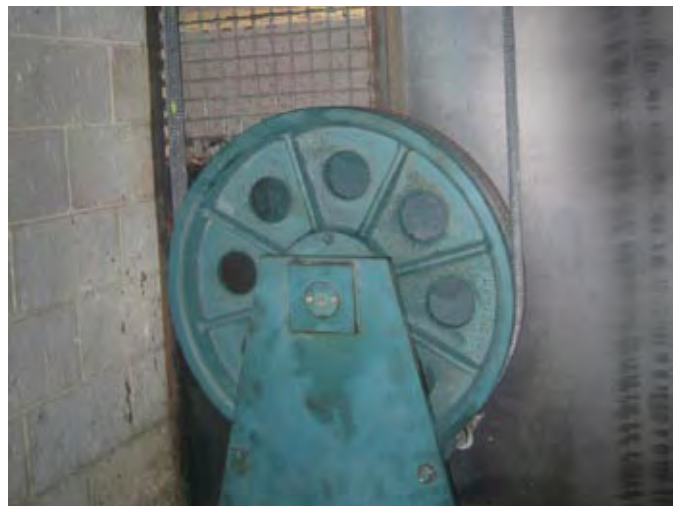
Fig. 15 AP bearings shown on typical elevator sheave application
